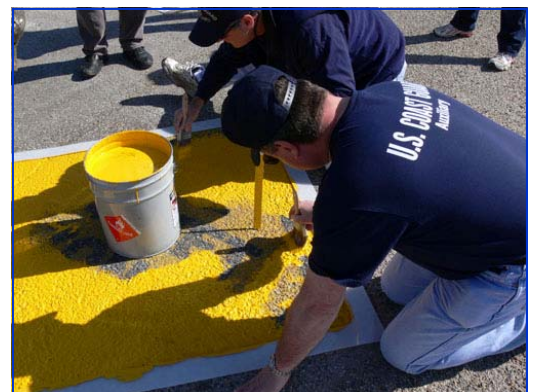
Auxilarists Wendy Faganel (above) and Phil Patterson (below) paint the yellow base for a "Life Jacket Zone" sign at Big Creek State Park. (U.S. Coast Guard Auxiliary Photo / photo by Suzanne Tomlinson)
